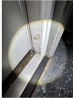
Basement doorway-bottom corner
