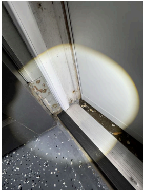
Basement doorway-bottom corner
