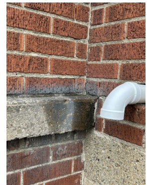
Right side of porch
