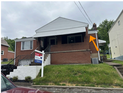
Right side of porch
